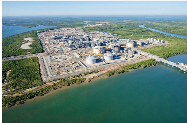
Plant overview of the INPEX-operated Ichthys LNG onshore processing facilities, in Darwin Australia.
