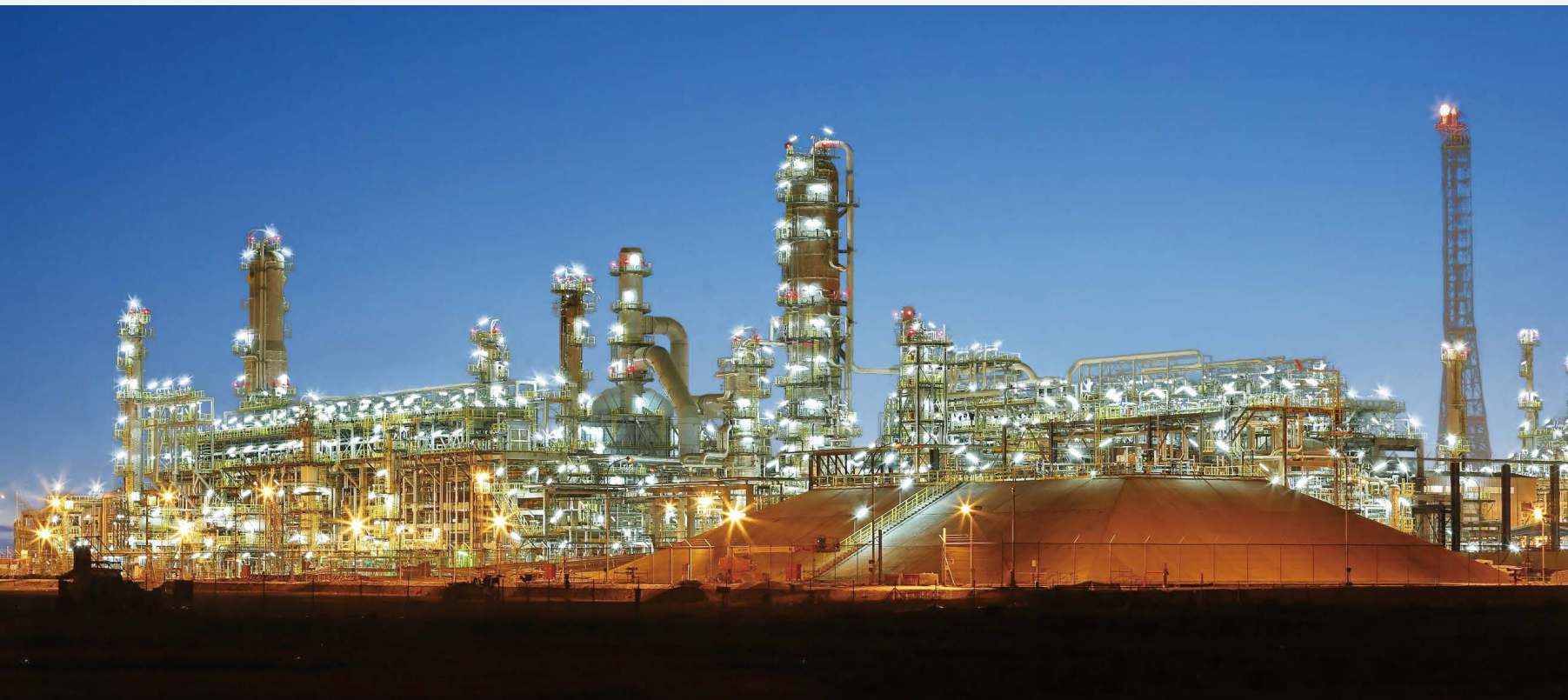
Laffan Refinery (Qatar)
