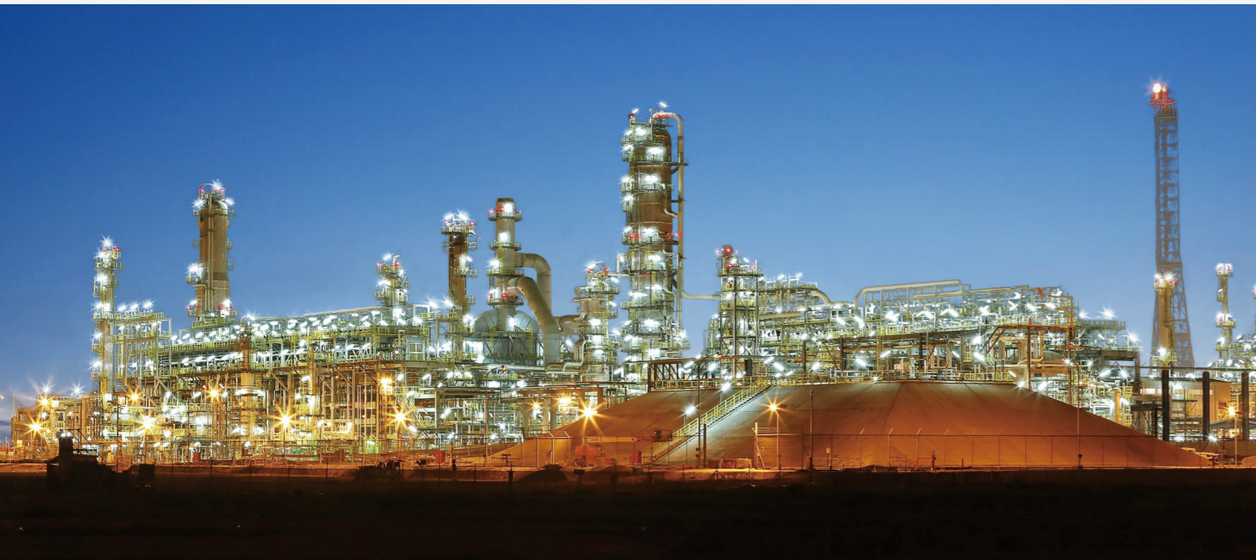
Laffan Refinery (Qatar)
