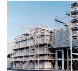
Flue Gas Desulfurization Plant (CT-121)(Japan)
