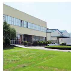
Food Factory (Modernized improvement)
