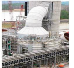
Flue Gas Desulfurization Plant (CT-121)(USA)
