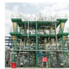
Demo Plant for SPERA Hydrogen
