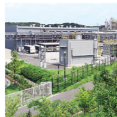
Refining and recycling of precious metals plant
