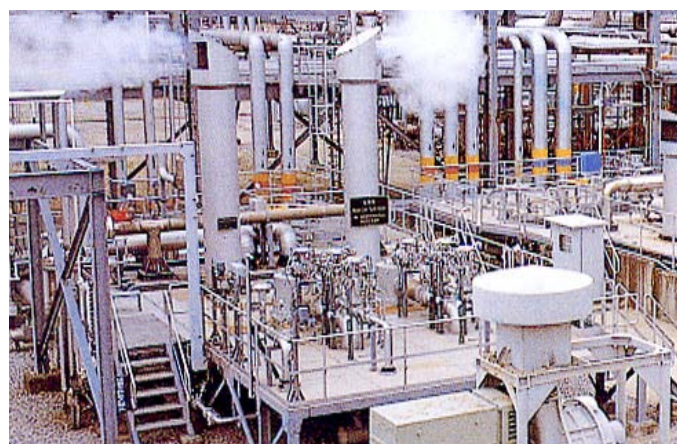
Submerged Combustion Type Vaporizer (SMV)
