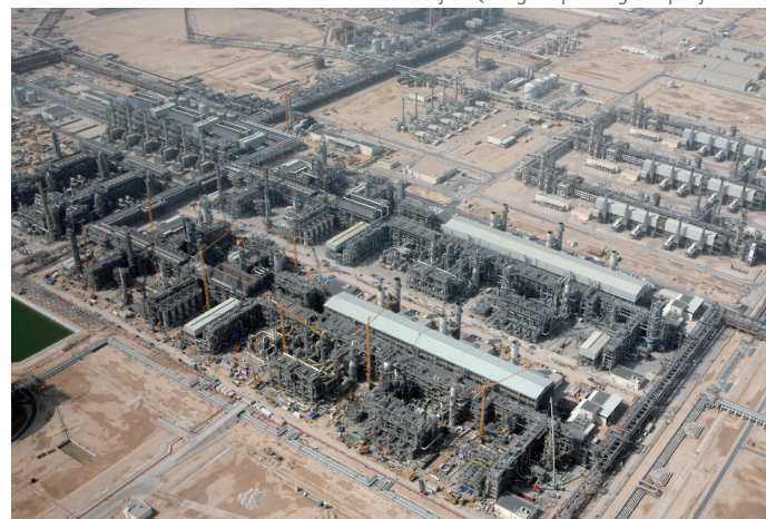
The World's Largest LNG Trains in Qatar
