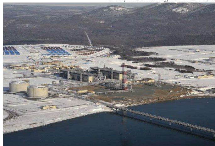
Execution in the harsh environment in Sakhalin Island
