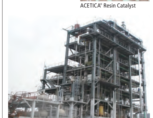
ACETICA® Demonstration Plant (36,000 T/Y)
