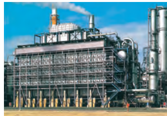
68,750 Nm³/Hr H₂ Plant
