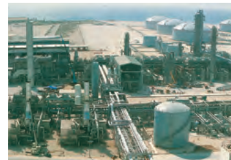
2,500 T/D Methanol Plant
