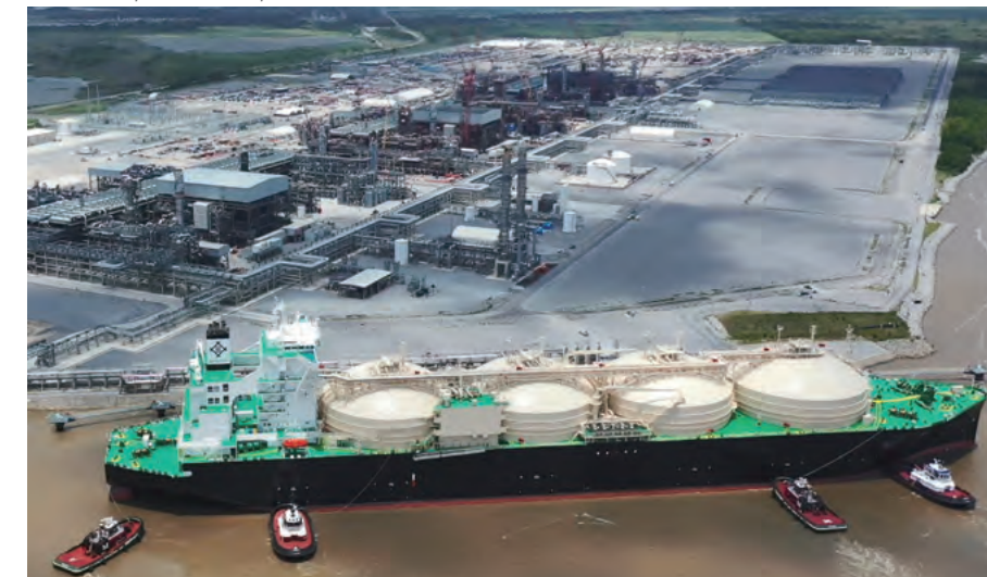
Cameron LNG, Louisiana State, USA
