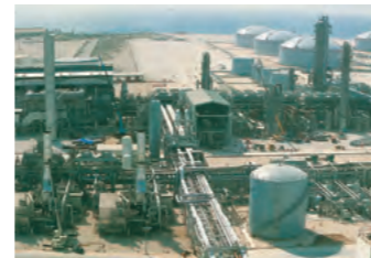
2,500 T/D Methanol Plant
