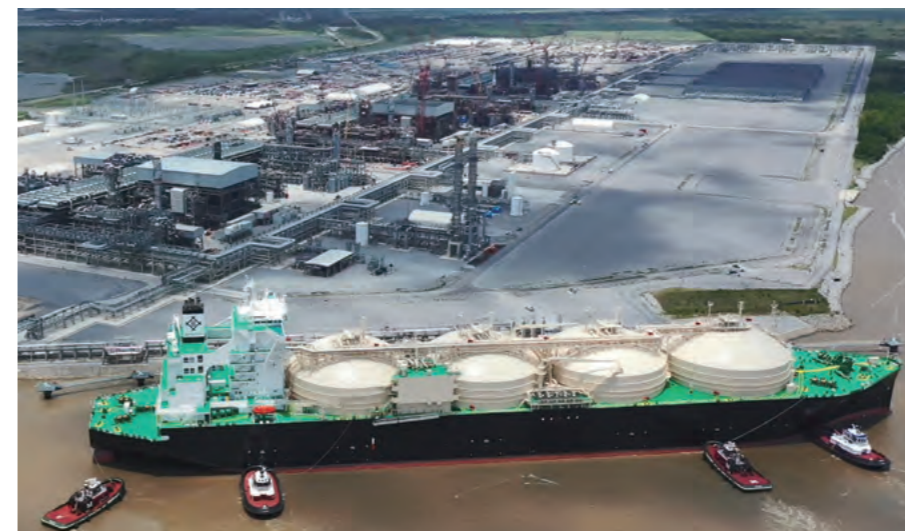
Cameron LNG, Louisiana State, USA
