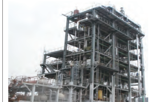
ACETICA ® Demonstration Plant (36,000 T/Y)
