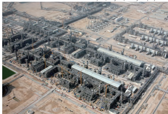
The World's Largest LNG Trains in Qatar
