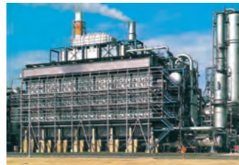
68,750 Nm 3 /Hr H 2 Plant
