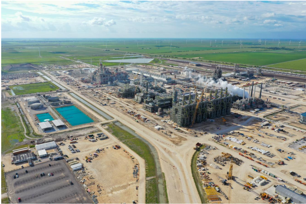
New petrochemical complex @ Texas.
