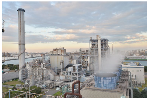
Hydrogen is supplied to Gas Turbines (Courtesy of TOA OIL CO., LTD.)
