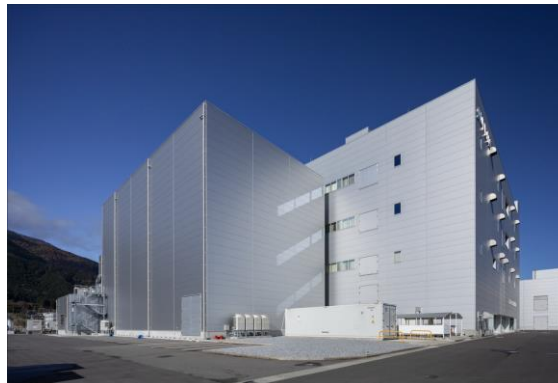
SHIONOGI & CO., Ltd. Vaccine Constituent Production Facility
