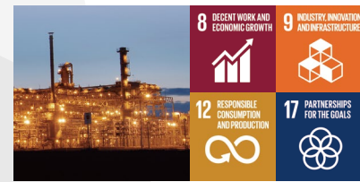
Plant Construction & Providing Infrastructure
