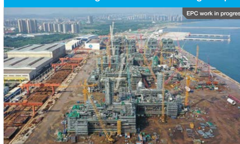
Overview of ongoing module fabrication
