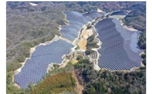
Pacifico Energy’s Toyota Mega Solar Power Plant
