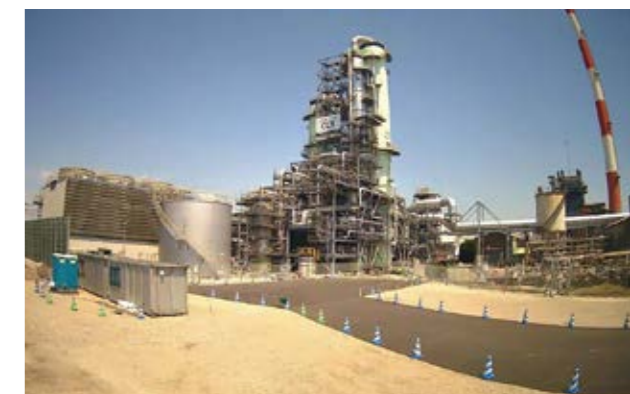
Construction of CCS demonstration plant
