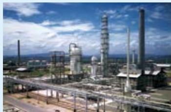
1960 Mitsubishi Oil Co., Ltd. Secured an order for Mizushima grass-roots refinery
