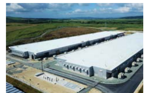
Construction of North Hokkaido Wind Energy Transmission Corporation’s storage battery system
