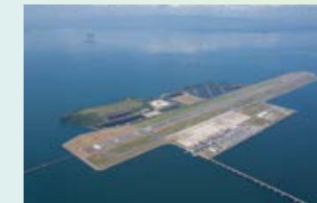
2011 Secured order for Nagasaki Solar Energy Co., Ltd.
