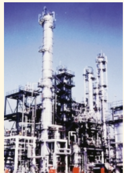
In January 1999, Chiyoda completed the construction of a benzene reduction facility at the Yamaguchi Refinery of Seibu Oil Company Limited.
