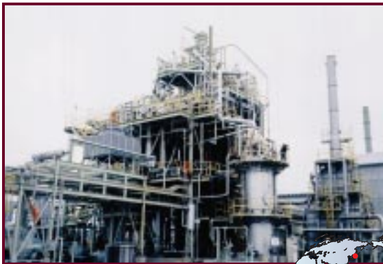
The Niigata Plastic-to-Oil Conversion Center has the capacity to convert 6,000 t/y of waste plastic into oil for use as fuel in public facilities.
