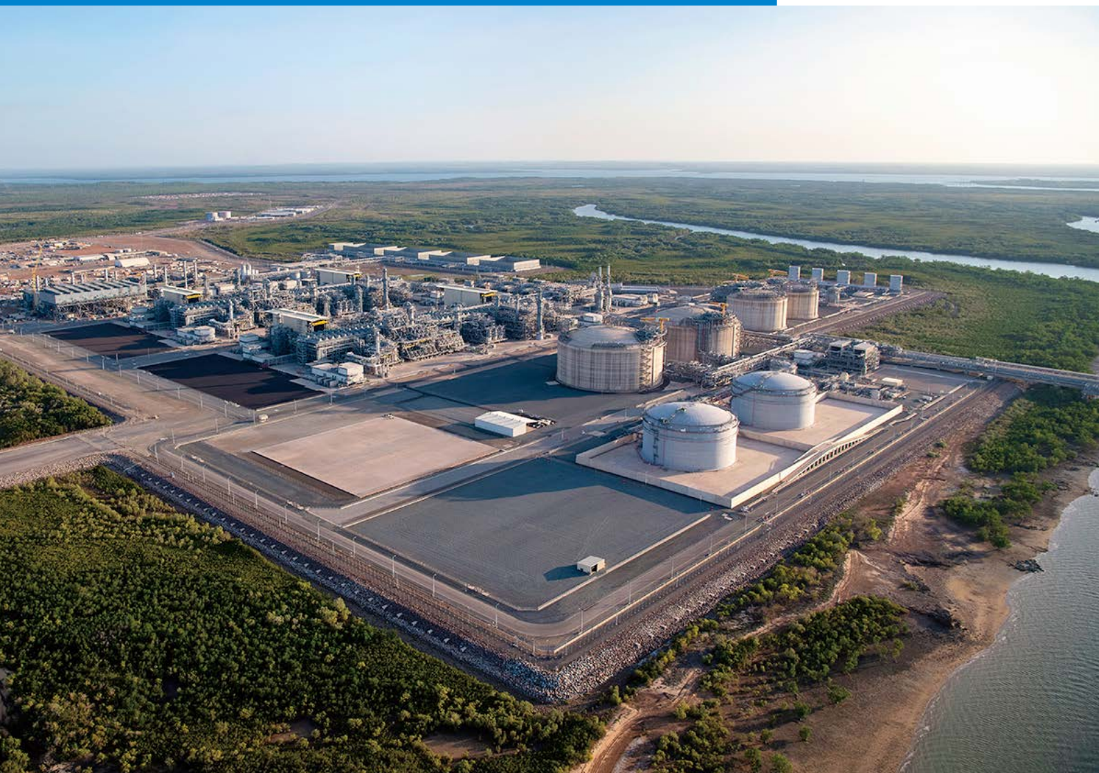
Photo courtesy of INPEX: Ichthys LNG Onshore Processing Facilities at Bladin Point near Darwin, Australia
