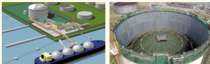
(Left) Artist's conception of completed LNG facility (Right) Inside of a LNG tank when empty
