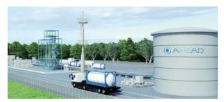
Hydrogenation Plant (Brunei Darussalam) In the supply country, hydrogen, chemically fixed to toluene, is converted into methylcyclohexane (MCH) by hydrogenation reaction for storage and transport.
