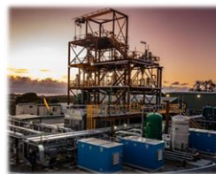
Demonstration plant currently under construction (Courtesy of Hazer)
