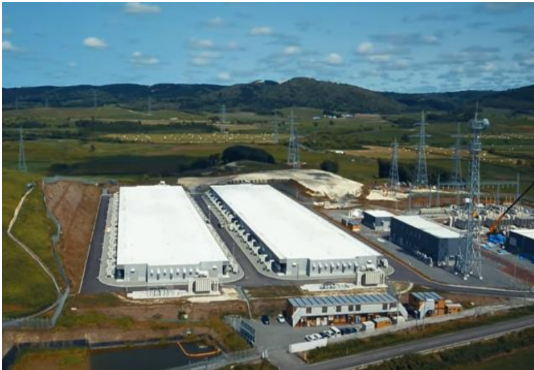
Energy Storage System Facility
