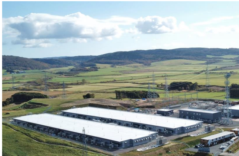
Energy storage system construction site
