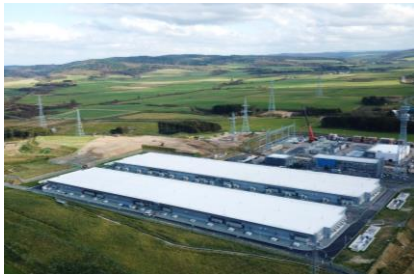
Battery power storage system (720MWh) EPC by Chiyoda (October, 2020)
