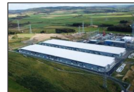
Storage battery system for North Hokkaido Wind Energy Transmission Corp.
