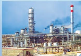
Petromin-Mobil Yanbu Refinery, Saudi Arabia
