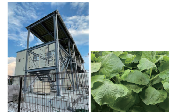
Plant Biofoundry Pilot Facility and Plants Under Cultivation
