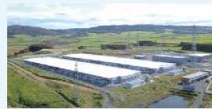
Storage battery system for Hokkaido Kita Wind Power Transmission Co., Ltd.
