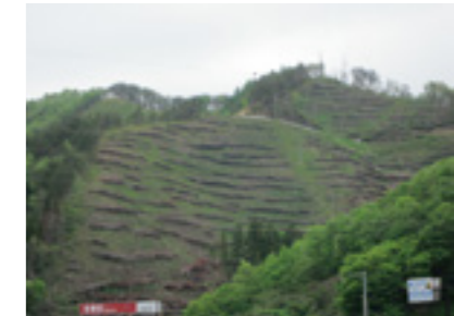
Mountain surface damaged by bushfires
