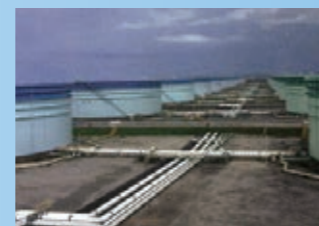
Complete construction of Fukui national petroleum stockpile base
