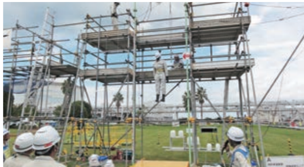
Simulated Experience Training at Oita Rinkai Field Office of Oita Liquefied Natural Gas Company, Inc.
