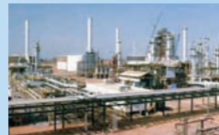
Kaduna refinery for NNPC (Nigeria)
