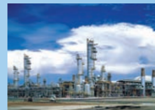
Arun natural gas liquefaction plant for Pertamina (Indonesia)
