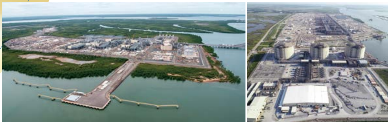
Ichthys LNG Project onshore processing facilities at Bladin Point, Darwin. Photo courtesy of INPEX Large Liquefaction Project Located in Louisiana USA
