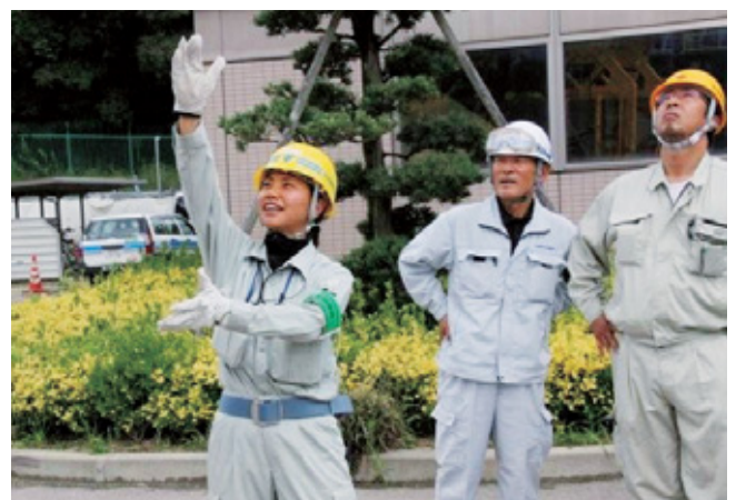
Women are active at plant construction sites.
