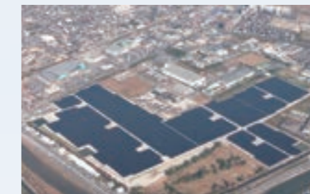
Photovoltaic power generation facility for Mitsui & Co., Ltd.
