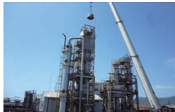
Scene of reconstruction work
