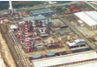
Copper smelter for P.T. Smelting Co.
