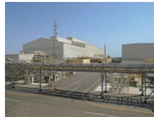
The completed sponge titanium manufacturing plant
