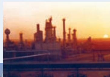
Riyadh refinery for Petromin (Saudi Arabia)
