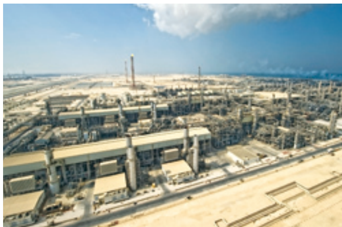
An LNG plant in Qatar, one of the world's largest with two trains that are each capable of producing 7.8 million tons of LNG annually (Photo courtesy of Qatar Gas Operating Company Limited)
