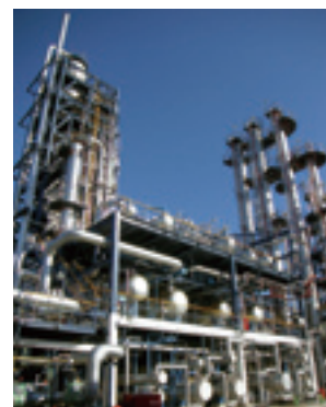
The HS-FCC Plant at Mizushima Refinery of JX Nippon Oil & Energy Corporation (Photo courtesy of JX Nippon Oil & Energy Corporation)
