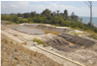
Onsite sedimentation pond
