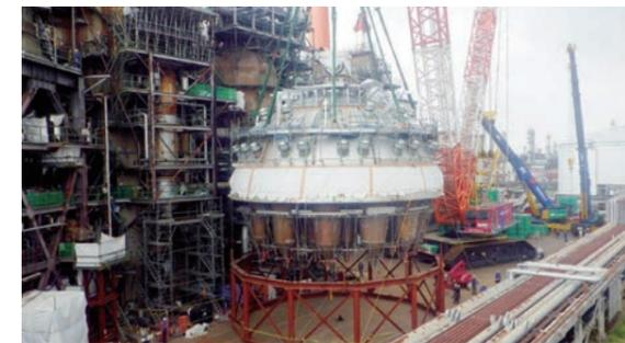
Column top portion of 16-m diameter regenerator that is largest in Japan
