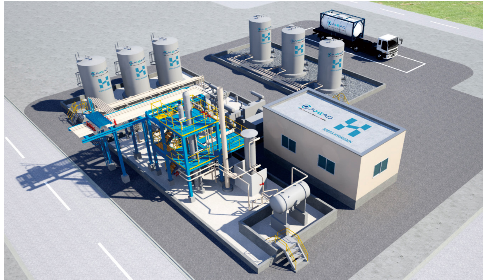
The Dehydrogenation Plant in TOA OIL's Keihin Refinery, Kawasaki's Rinkai Industrial Area and Port (Japan)
