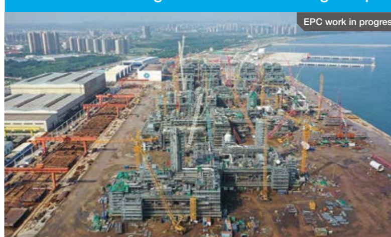
Overview of ongoing module fabrication
