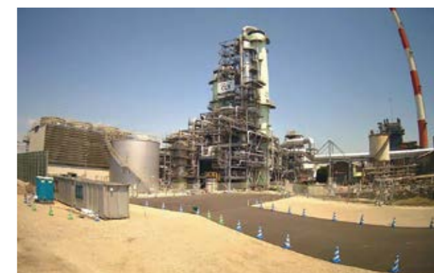
Construction of CCS demonstration plant
